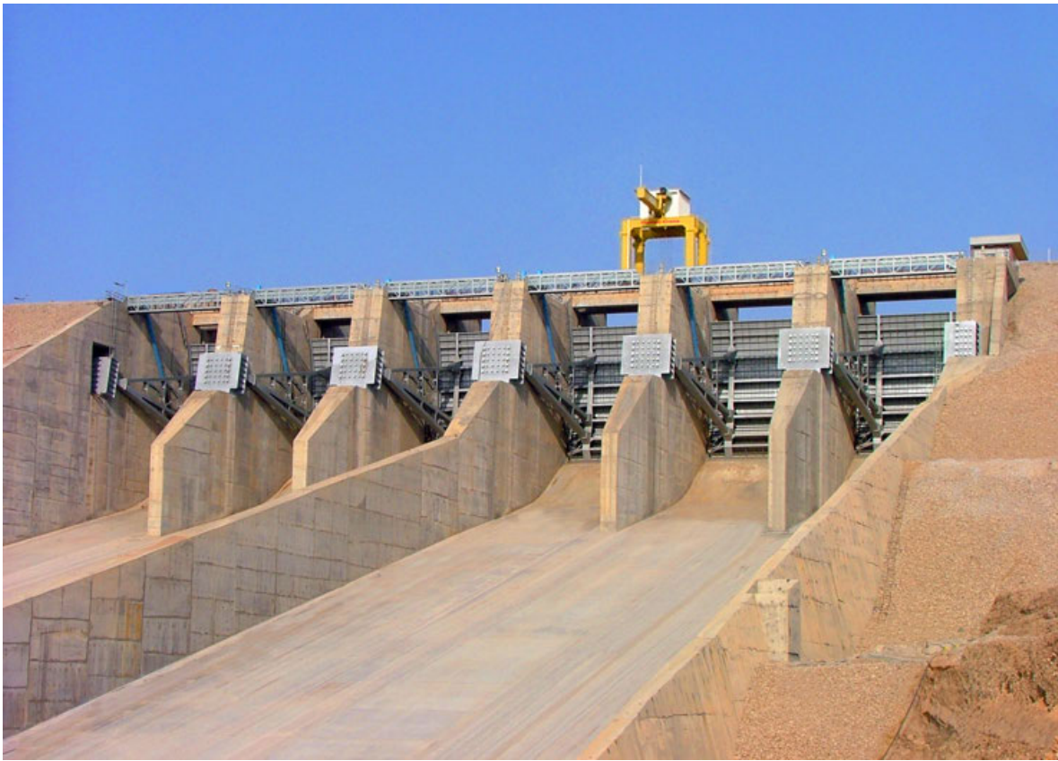
Dam Crane –Gantry Crane 40/3.2 Ton – with 8 meters outreach access for gate maintenance
