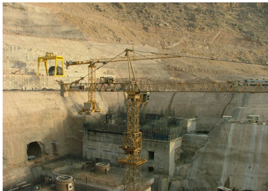
Dam— Gantry Crane 40/5 Ton with 50 meters lifting height for installation of the pipes of dam.
