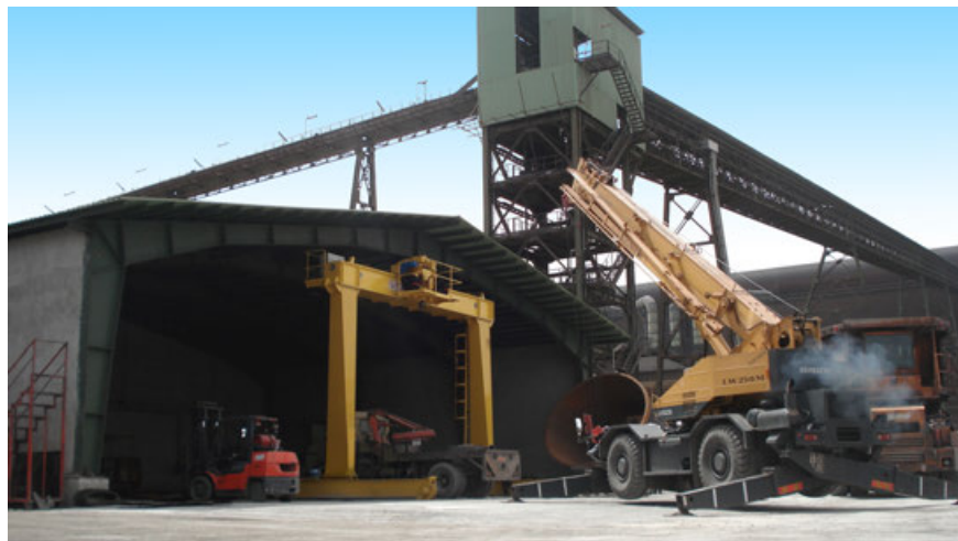
Steel Making Plant Ladle Maintenance Workshop Multi-Purpose Gantry Crane
