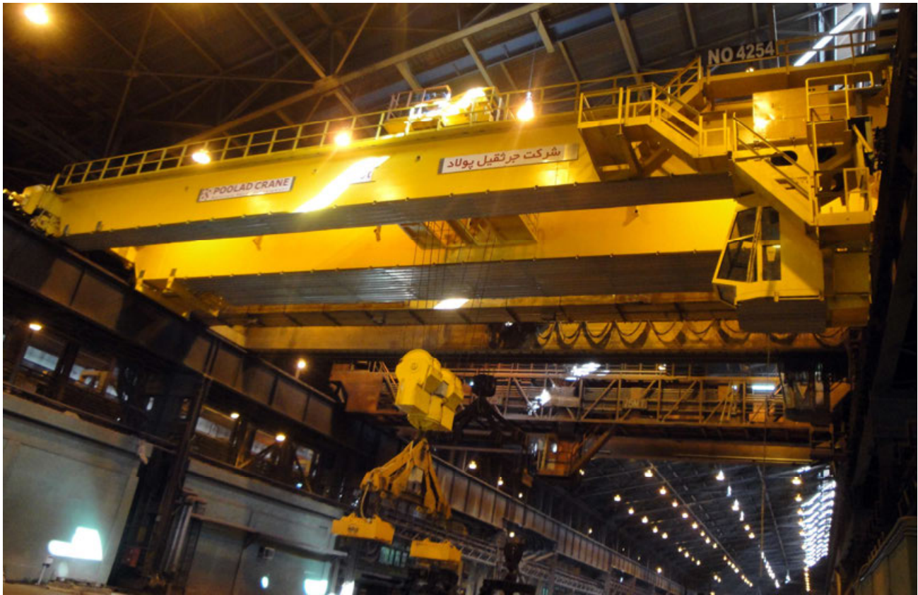
Steel Making Plant – Billet Bay Crane – FEM Classification A8 M8
